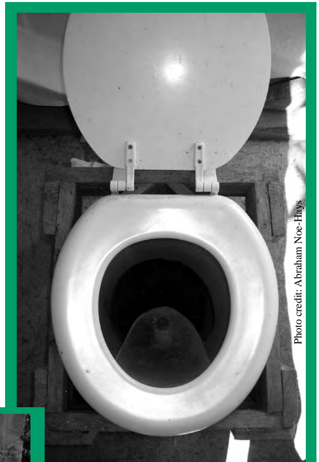
Above: Urine diverter made from a plastic soda bottle fits under the seat of the dehydrating ecosan latrine at Honduras Demo Farm.
